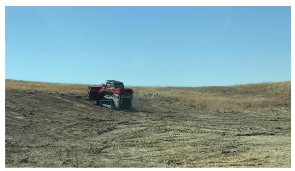
Figure 4: A skid steer with a till attachment was used to till the reclaimed sinkhole areas.
