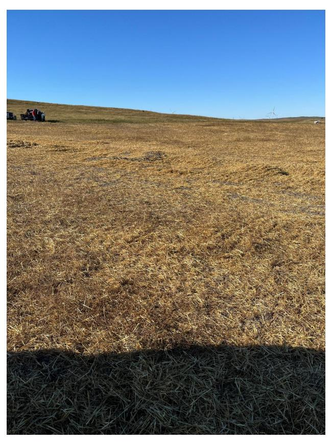
**Figure 14:** Erosion features were graded, and straw mulch was crimped to prevent further erosion.
