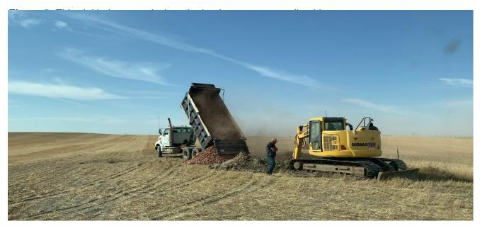
**Figure 6:** This sinkhole is being filled with scoria and soil from a nearby borrow location provided by the landowner.
