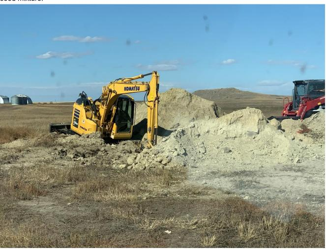
**Figure 2:** When the excavator opened up this sinkhole, the mine void was more than twice as large as expected.
